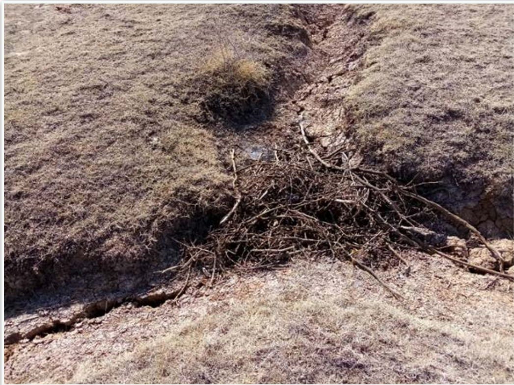
Figure 86. Junction of infiltration canals with a high-flood mark.
